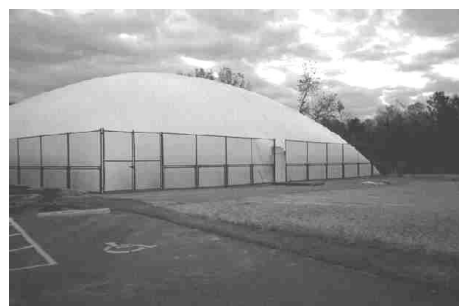
Fig. 4. Roof over tennis court
