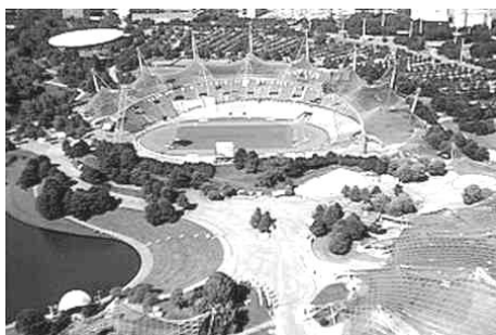
Fig.2. Olympic stadium roof in Munich
